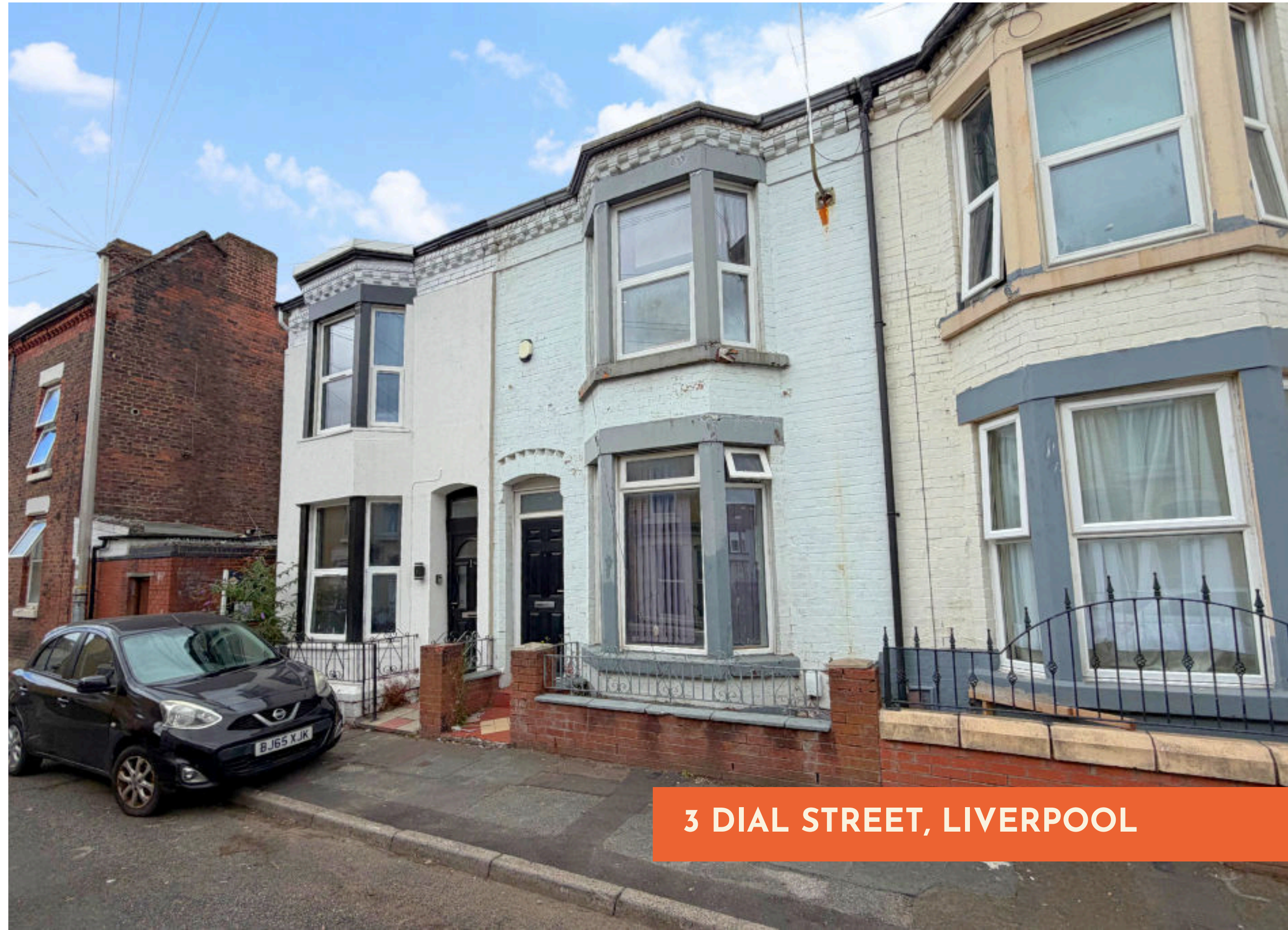
FRONT OF BUILDING
